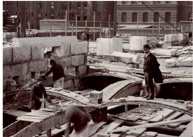
Fig. 3. Guastavino standing up on a newly built arch during the construction of the Boston Public Library, 1889. (Image courtesy of Boston Public Library, “Boylston Street” August 31, 2006 via Flickr, Creative Commons Attribution).
