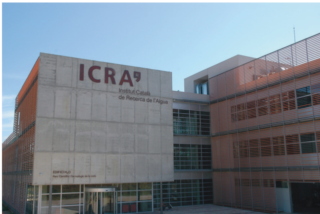
Fig. 1. External view of the ICRA's H2O building.
