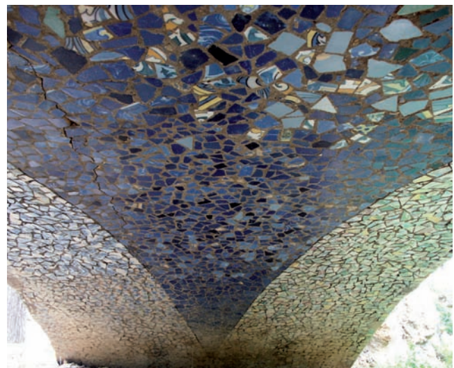
Fig. 21. Bottom surface of the Cova Cascada bridge; it can only be seen reflected in the water (1907).
