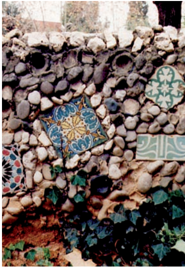
Fig. 6. Back of one of the trencadis benches, set with pebbles and pieces of broken tiles and glass bottles (1912).
