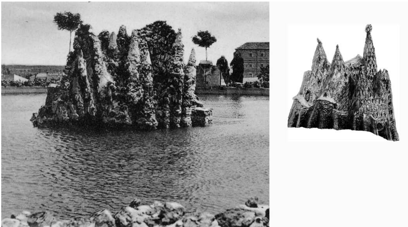
Fig. 22. Montserratina structure, located in the middle of the water reservoir of Sant Boi Mental Hospital. According to the journal Revista Frenopàtica Española , this reservoir was built in February 1910. It also appears duplicated as “Detail A” in a plan published by Miquelerena [1] (postcard from the beginning of the 20th century; from the collection of the author). The structure directly resembles a drawing of the Colònia Güell church published by Gaudí in the same year.
