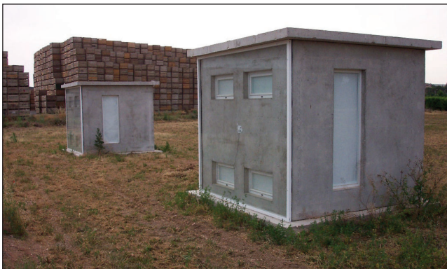
Figure 8. View of the cubicles with Trombe wall.
