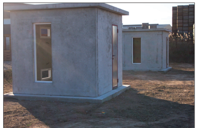
Figure 5. View of the cubicles.
