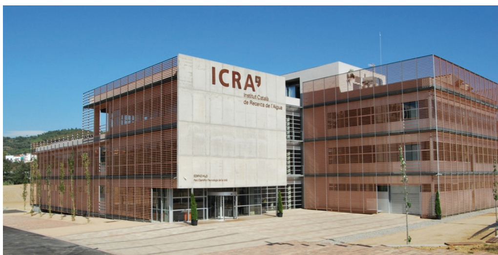
Fig. 1. The H 2 O building of the Catalan Institute for Water Research (ICRA), Girona.
