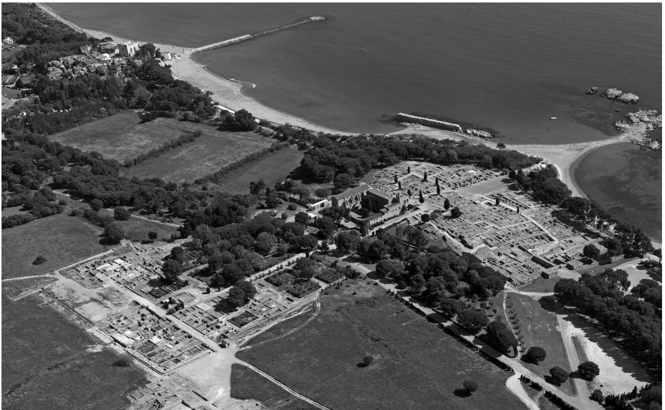
FIGURE 1. Aerial image of Empúries. Above left, the current nucleus of Sant Martí d'Empúries, located over the remains of the first establishment of the Palaià Polis . On the right, separated by the hollow of the ancient natural port, the Neapolis sector, the main urban nucleus of the Greek city of Emporion (Photo: MAC-Empúries. S. Font).
