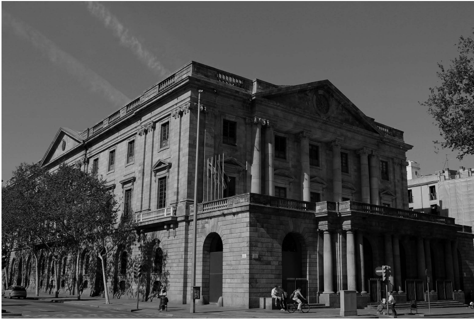
Figure 4. The building housing the Board of Trade of Barcelona, which created technical schools and chairs aimed at sharing European scientific advances. The outside is neoclassical in style and was built in the last third of the 18th century, while the interior, which is Gothic and dates from the 14th century, is the sea exchange.
