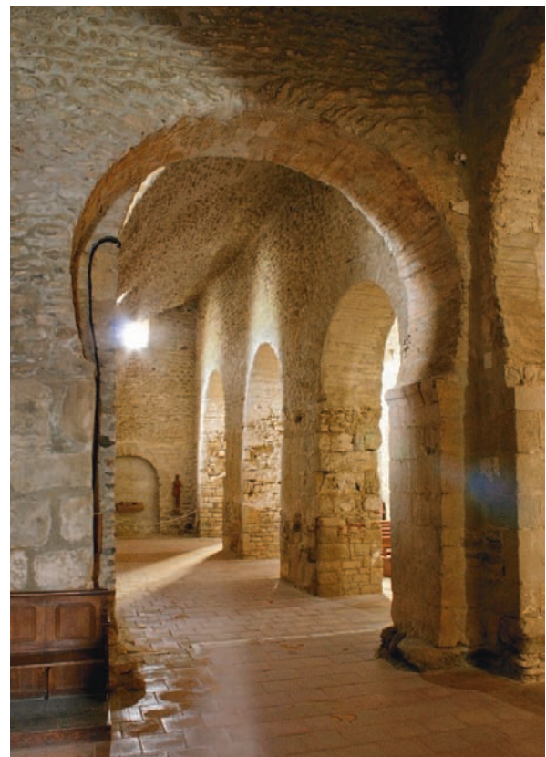
Figure 4. View of the southern side nave in Sant Miquel Cuixà from the southern wing of the transept. The ultra-semicircular arches can be seen.
