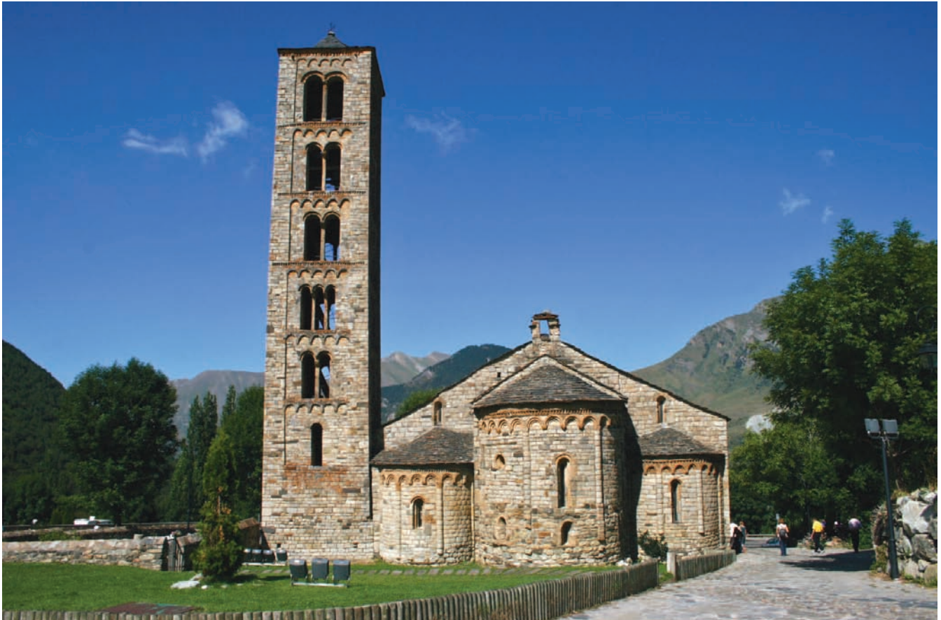
Figure 1. Romanesque church of Sant Climent de Taüll. It shows a basilica layout with three naves, an apse and two apsidioles, plus a tower on the southern facade facing east very close to the apse. The belfry is square and freestanding, although it is built very close to the bulk of the building on the corner of the southern wall next to the chevet. Photo: Jesús Cano Sánchez.
