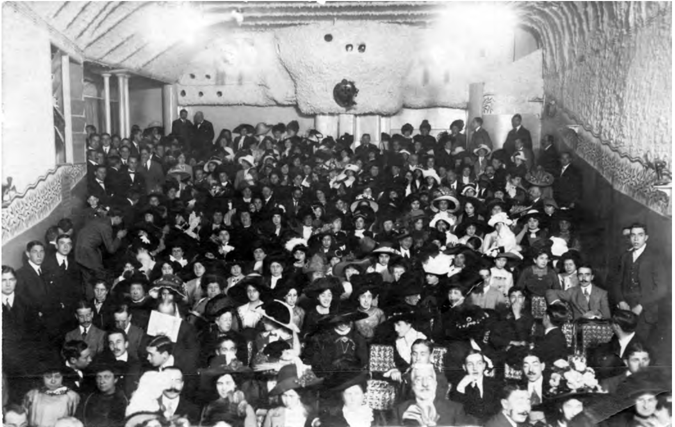
FIGURE 6. Interior of the Sala Mercè. Barcelona. Photo: author unknown (1910-1912). GMN Archive.
