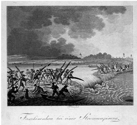
Figure 5. Constructing Faschinen .
