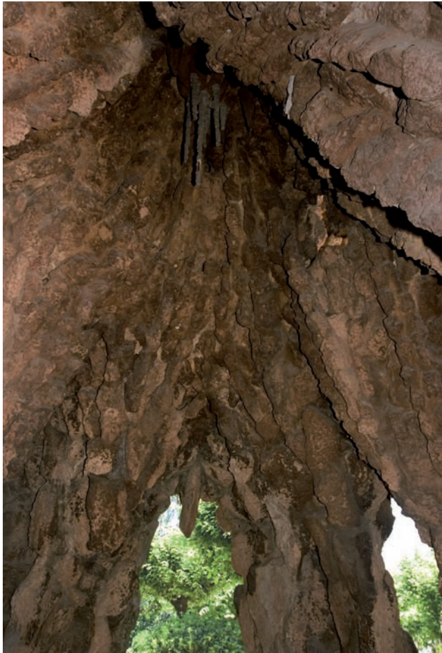
Fig. 10. Main vault of the Cova Cascada.
