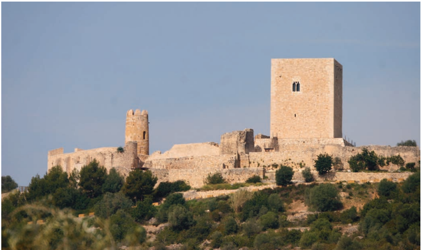
Figure 6. Ulldecona Castle. It was part of the Catalan frontier with the Saracens until the Valencian campaigns of James I starting in around 1230. Today, you can see a walled area with a round tower with Arab origins and the palace tower of the Order of the Hospital. The square-shaped building features a semicircular arched window. Photo: Jesús Cano Sánchez.
