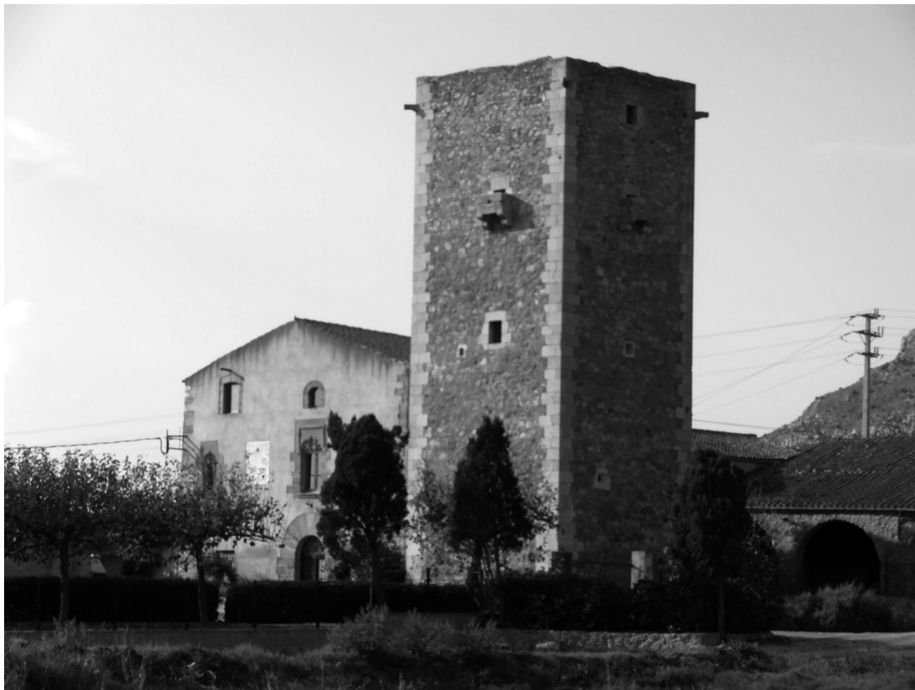
FIGURE 3. Torre Bagura farmhouse (Torroella de Montgrí, photograph by J. Serra), where the tower was built in the second half of the 16th century. In the photograph, note the farmhouse with three bodies, three storeys, voussoir door and carved window. This is a prototypical farmhouse from the late 16th century.
