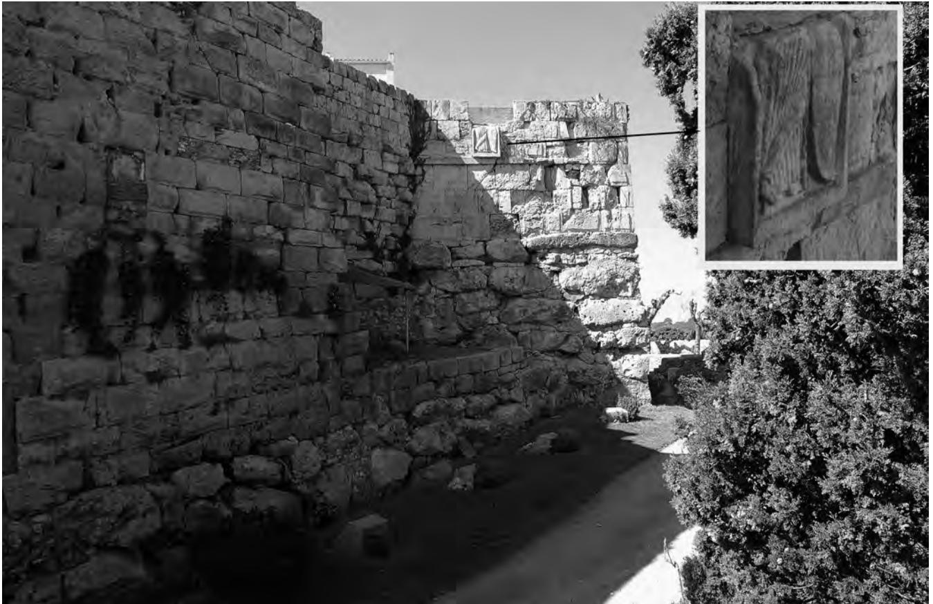
FIGURE 2. Minerva Tower sector; detail of the relief and two building techniques (photo: J. M. Macias).
